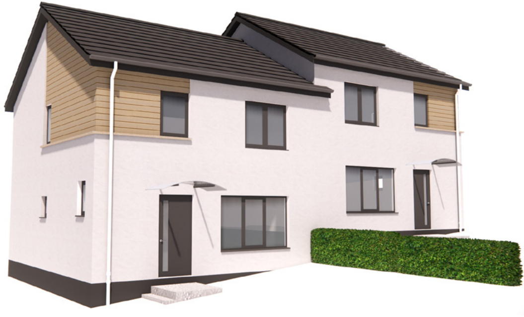
House B2 MacRobert stepped frontage
